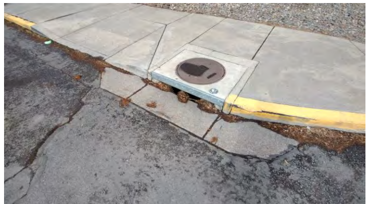
Curb inlet in the neighborhood
