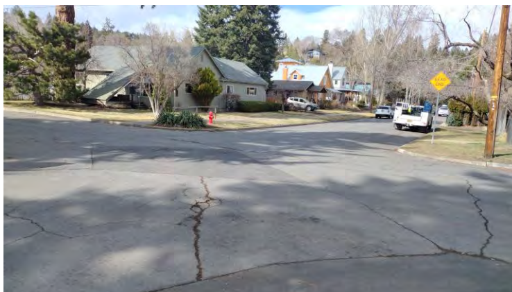
Intersection of NW Saginaw Ave & NW 1 st St, looking northwest
