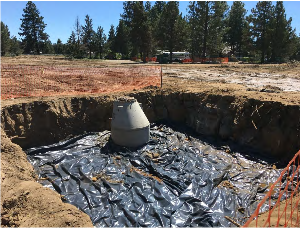
Figure 18. 6-mil plastic sheeting installed prior to concrete pour.
