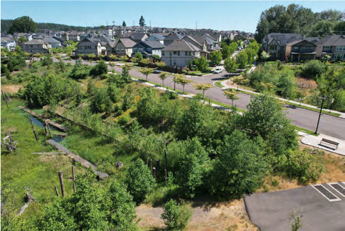
Figure 8. Aerial drone photograph of a regional stormwater quality and quantity control facility (bottom left) serving a large subdivision – including public roads and private parcels – in Tigard, Oregon.
