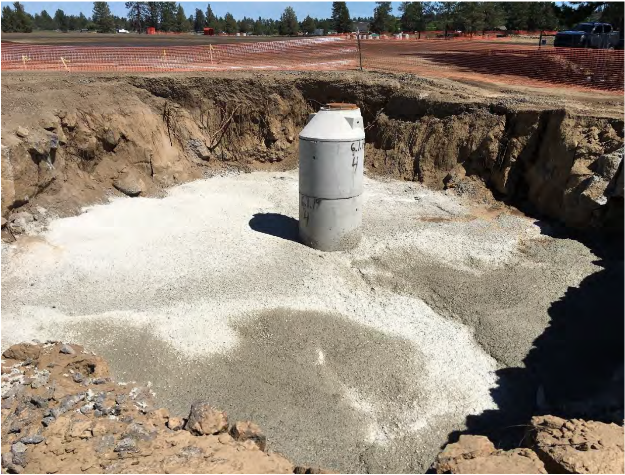
Figure 19. Concrete cap poured over plastic sheeting.
