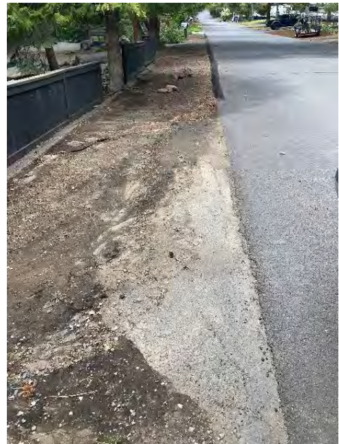
Runoff effect from asphalt curb
