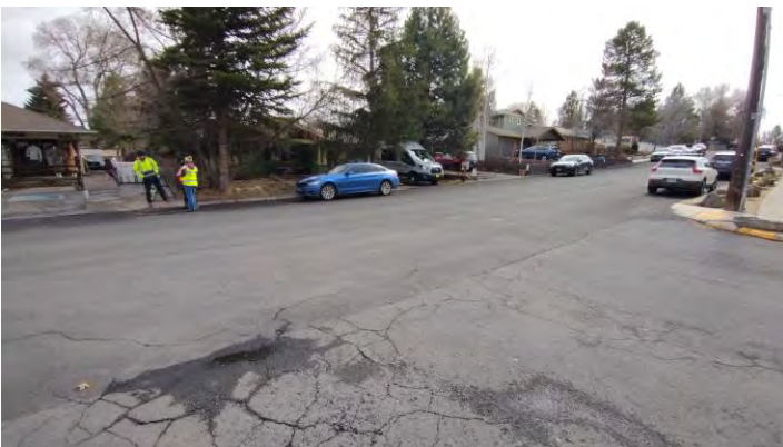
NW Fresno Ave & NW 12 th St looking southeast
