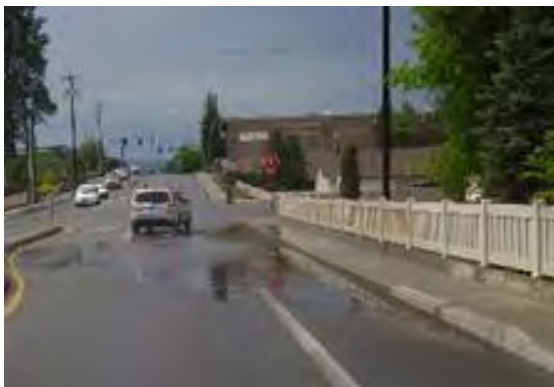
Ponding on NW Olney Ave impacting travel
