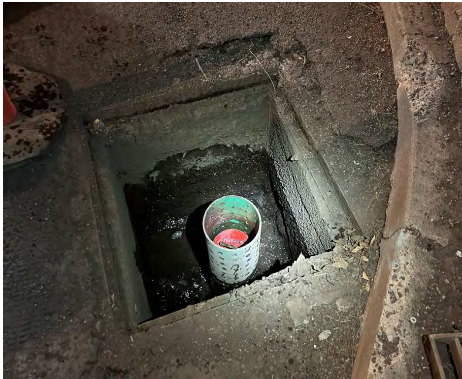
Figure 5. A typical drillhole in catch basin.
