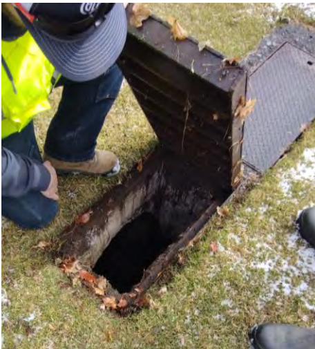
Storm facility access in Drake Park
