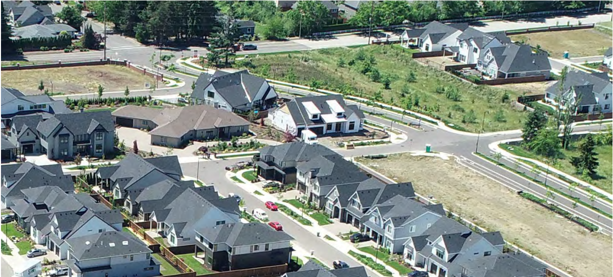
Figure 7. Aerial drone photograph looking southwest of the partially constructed subdivision phase showing detention pond in Tract G, examples of private rain gardens, and examples of vegetated swales serving public ROW.
