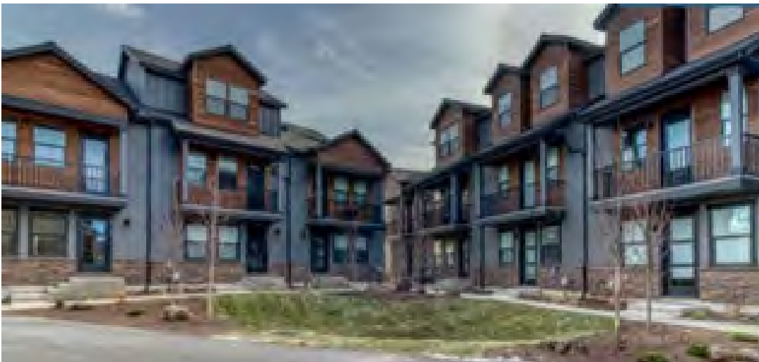
Figure 10. Photograph of a centralized stormwater facility at Calaveras townhome development near Empire Ave and Boyd Acres Rd
