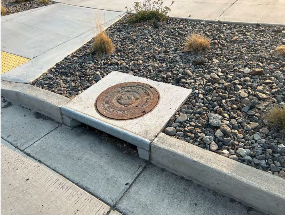
Figure 13. An Example of a CG3 Curb Inlet Catch Basin.
