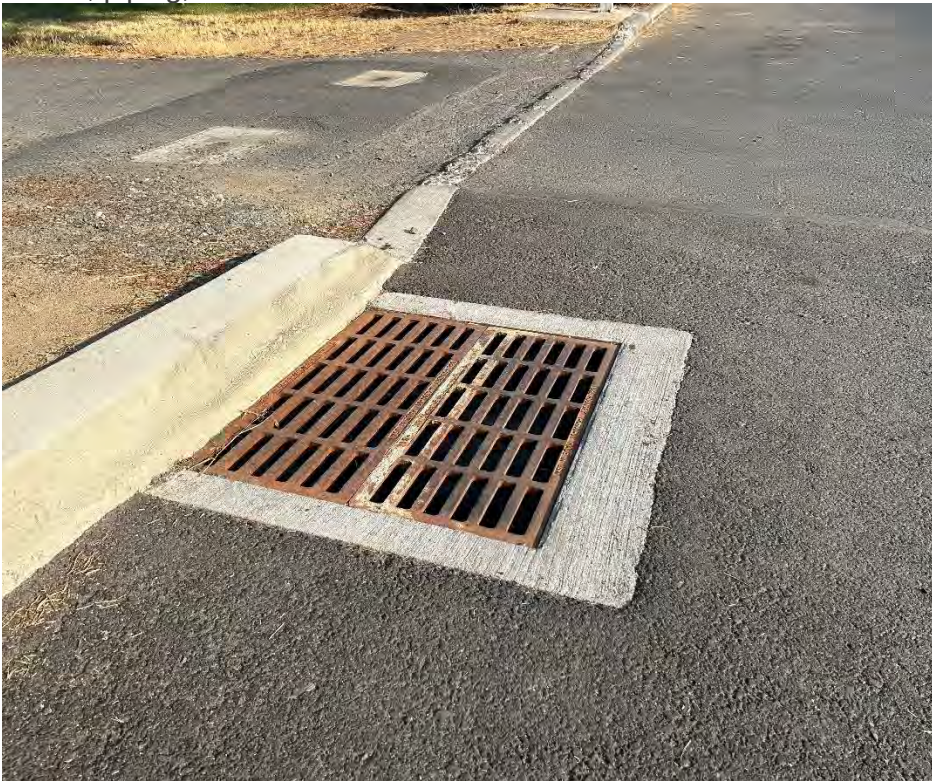
Figure 12. An Example of a G2 Style Catch Basin.
