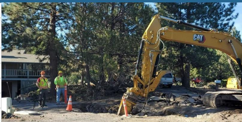
Sample Septic to Sewer photo showing excavation to install a service lateral to a property.
