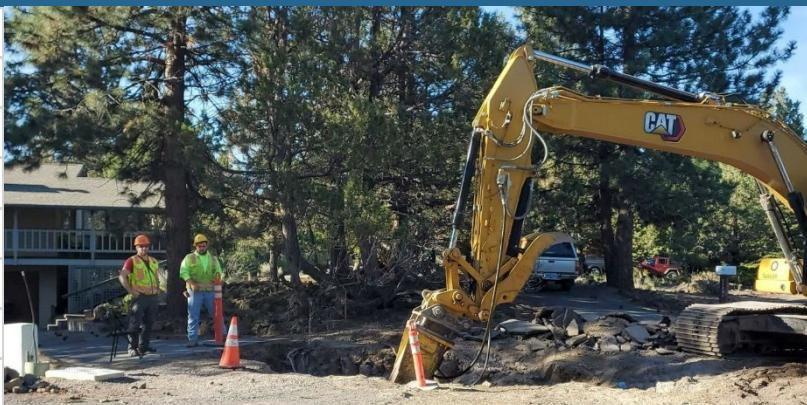
Septic To Sewer sample photo for installation of a sewer service lateral to a property.
