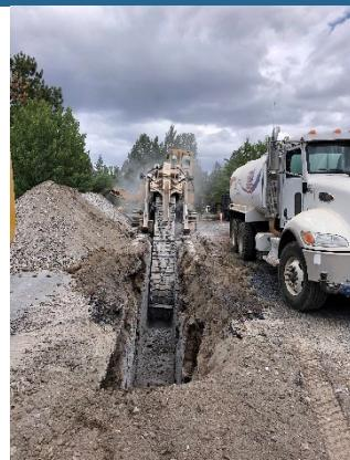
Rock-sawing for the sewer mainline trench on West View Drive.
