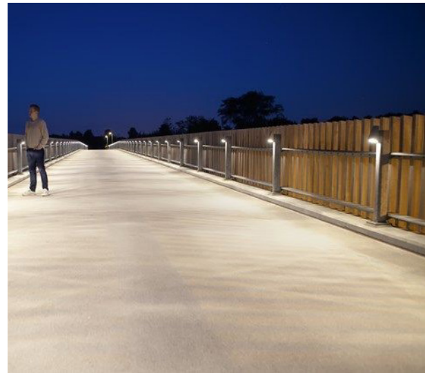
Intermittent Handrail Lighting
