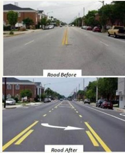
The image shows a two-part photograph of a street. The top part, labeled 'Road Before', shows a four-lane road with a double yellow line down the center and no turn lanes. The bottom part, labeled 'Road After', shows the same road with a dedicated left-turn lane on the left side of the center line, and the double yellow line is shifted to the right. A white arrow on the road indicates the direction of the left-turn lane.
