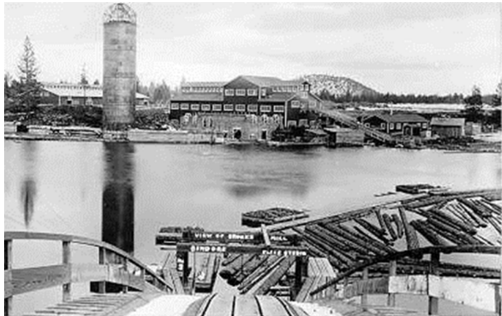
Figure 3-1. Shevlin-Hixon mill on east side of river as seen from Brooks-Scanlon mill
