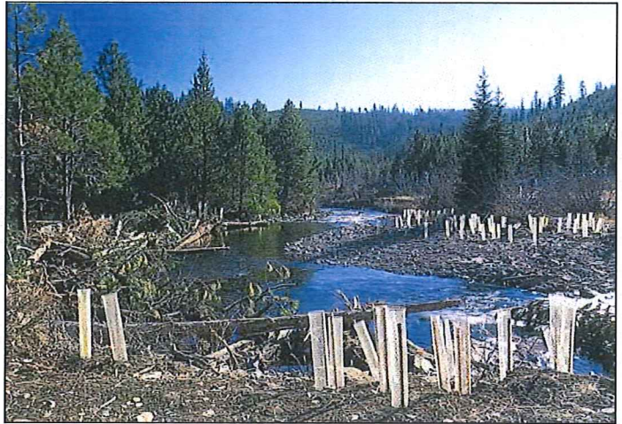
Throughout the 2.8-mile project area, restoration focused on improving fish habitat by increasing sinuosity, adding large woody material and planting native riparian vegetation.
