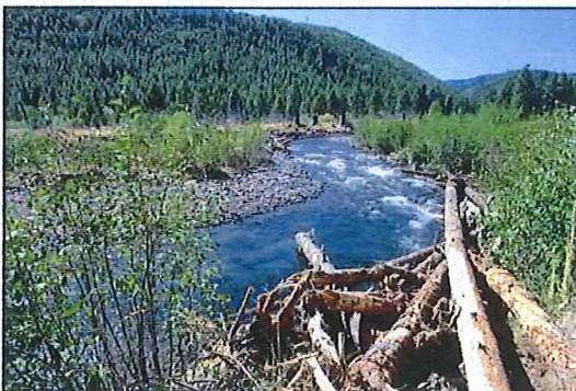
Created logjam structures (left) help increase bank stability, provide cover for fish and retain deep pools. The log structures are assembled from whole trees keyed into the creek banks to provide long-term bank stability (right).
