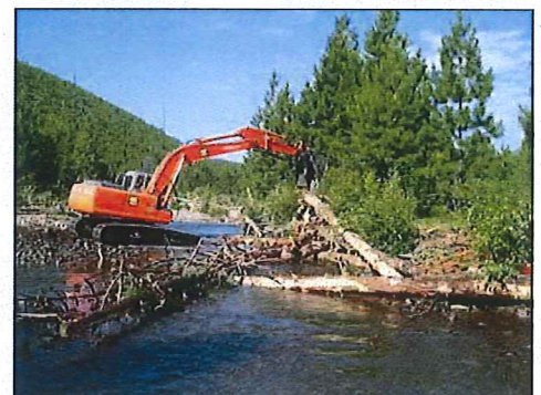
Created logjam structures (left) help increase bank stability, provide cover for fish and retain deep pools. The log structures are assembled from whole trees keyed into the creek banks to provide long-term bank stability (right).
